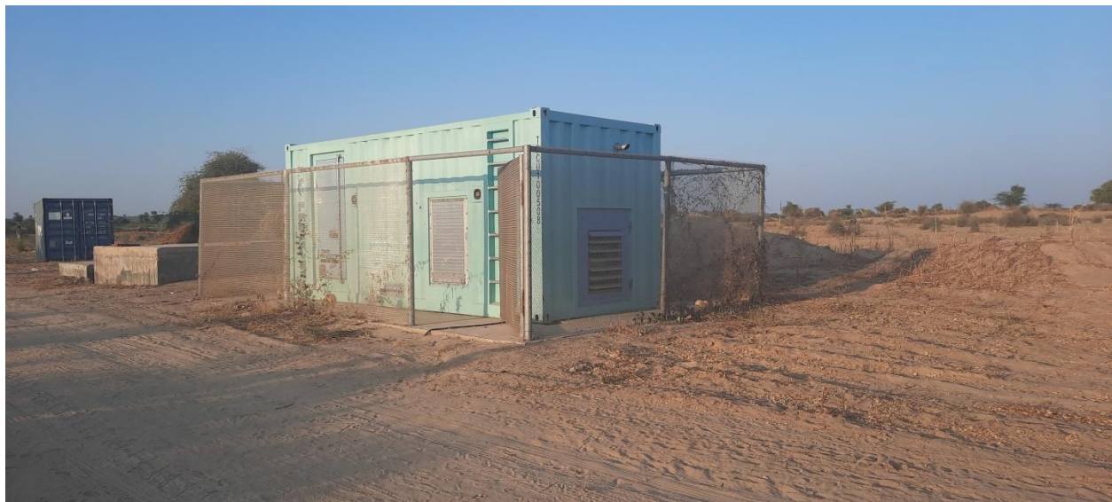
Mine water reinjection plant at Meghay Jo Tar village
