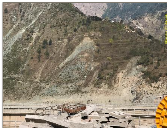
Figure 10: The dam is built right over an active fault. Right next to the dam is mountain face with a number of recent landslides due to fault movement
