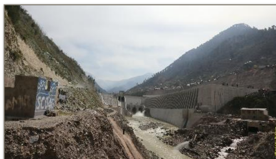
Figure 08: There is no passage for fish in the dam. The river has been fragmented.
