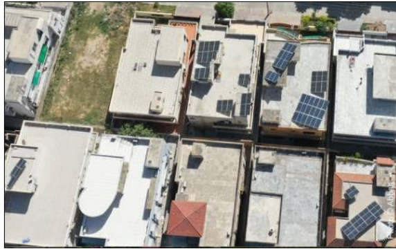
Figure 4: Rooftop solar PV in Sector E-11, Islamabad.
