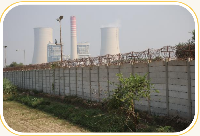
A view of the plant's outer boundary wall.
