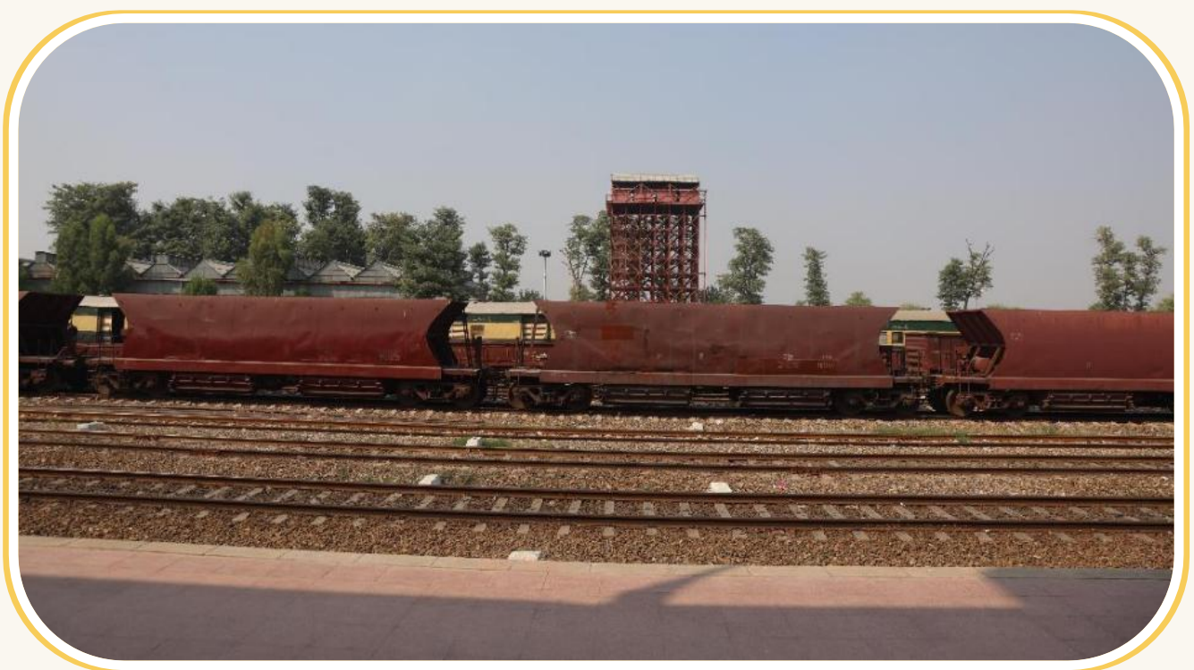
Yousafwala Railway Station was redesigned to serve the plant and is now closed to the public.
