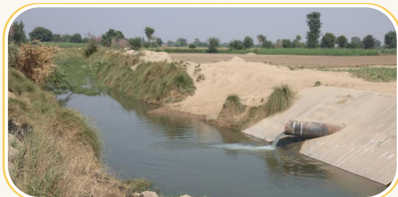
Discharge outfall pipe of waste water
